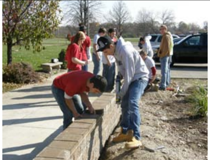
WCCC students at work on a retaining wall.
